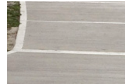
Brushed Concrete with trowel edge finish (streets)
