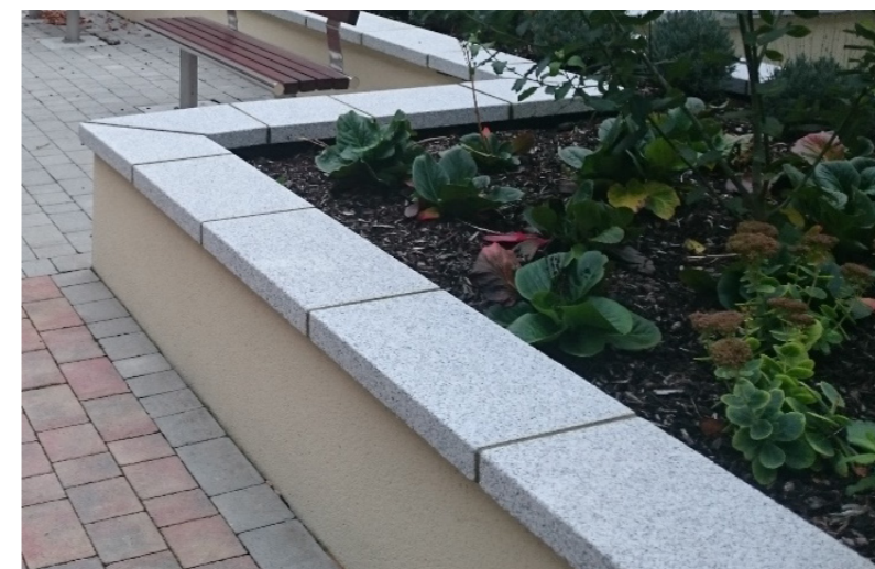
Planter/Vent Walls on Podium & Pedestrian Street
